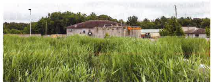
In 2015, the Mora Wastewater Treatment Facility received Clean Water Funds to construct upgrades that reduced phosphorus discharge to the Snake River by 74 percent.
